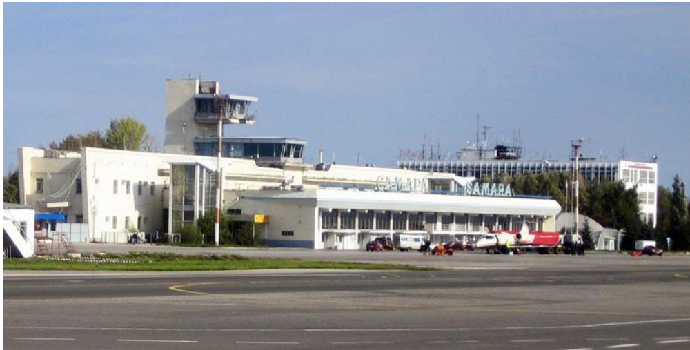
Kurumoch International Airport (Samara)
